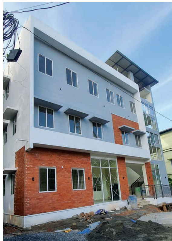
The new building for Perumbadappu Panchayath office
